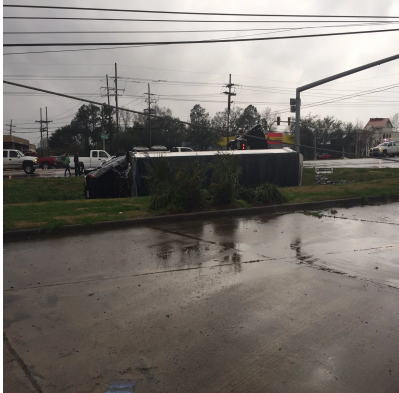
2016 LaPlace, LA Tornado Damage
