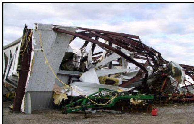
An EF3 tornado destroyed this shed in east central Noxubee County on New Year's Day 2011. Photo by NWS Jackson, MS
