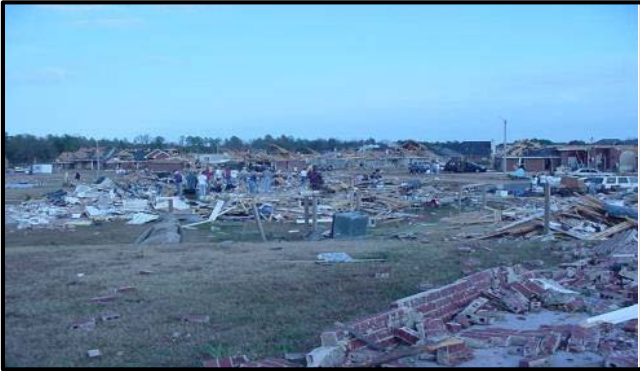
An F4 tornado caused significant damage to the Fairfield subdivision near Madison, MS on November 24, 2001. Photo by NWS Jackson, MS
