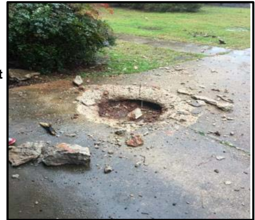
A lightning strike caused Extensive damage to this Driveway Photo by Chris Curlee
