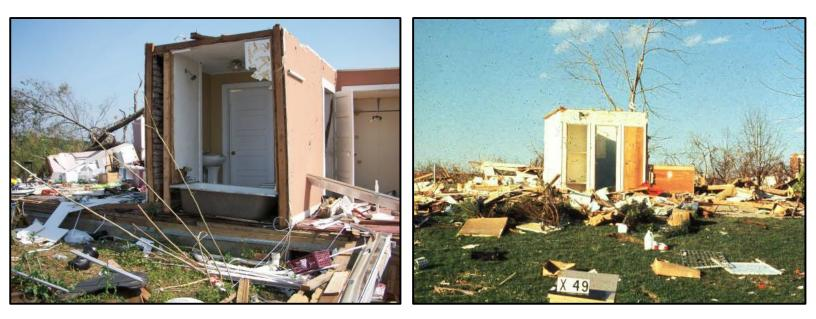
Outside walls of these homes collapsed after being struck by a tornado. Interior walls remain standing. Both of these photos show why being in the interior portion of a home/building is important, and why wearing a helmet is a good idea.
