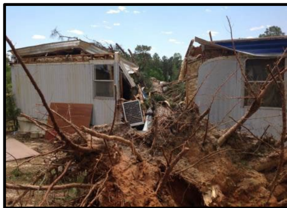
Straight-line winds in excess of 90 mph downed a tree through a mobile home in Wayne County on April 29, 2014. Photo by NWS Mobile, AL
